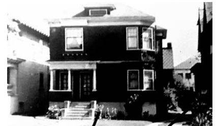
An affordable housing building demolished by UC in 1968. The people of Berkeley turned the vacant lot into a park.
